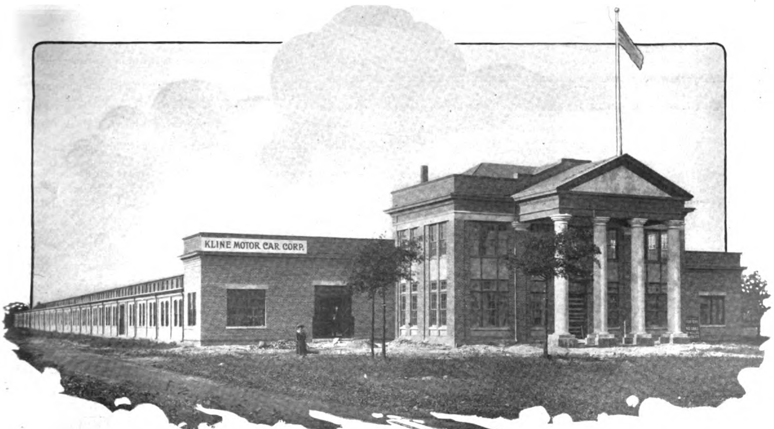
New factory of the Kline Motor Car Corporation at Richmond, Va., to which the company is now moving its machinery and equipment
